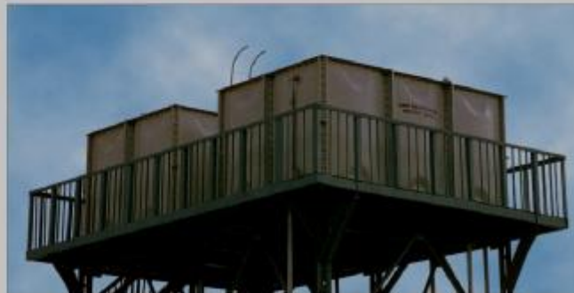
2m deep 2x12 KL tanks for Drinking water at an Educational Institute
