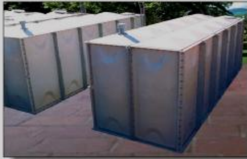
2m deep 24 KL tanks with 2x1m panel for drinking water storage at a Hotel in Kashmir
