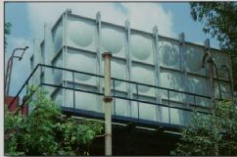
3m deep 54 KL tank for drinking water for a Housing Colony
