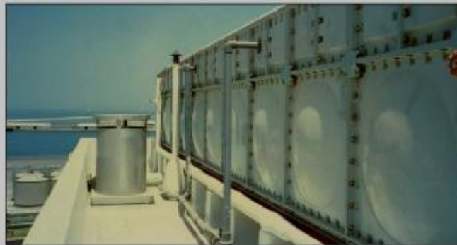
1.5m. Deep, PUF insulated panel tank for drinking water in KSA, with FRP skin for protection of PUF)
