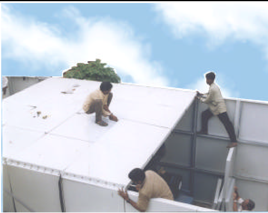
"Duro-STOR" modular housing system being assembled at site.
